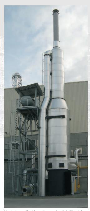
Heater in vertical layout, capacity: 9.6 MW with built-in combustion air preheater and subsequent stack, total height: 25 m, fired with natural gas; for heating of a particleboard press, Romania
