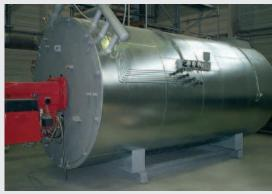
Thermal oil heater fired with natural gas with a capacity of 1.6 MW, installed in Texas, USA, for the food industry
